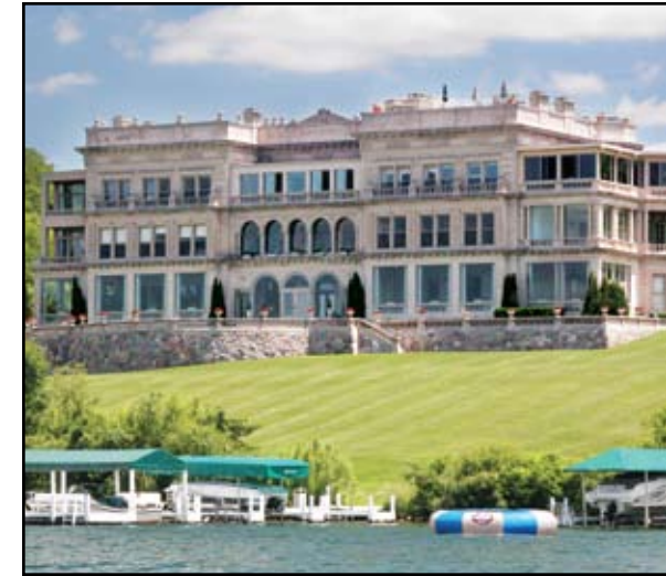
A view of the fifty-room mansion on Lake Geneva
